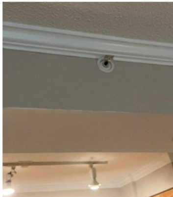
A residential fire suppression system installed throughout the home.
