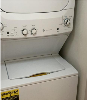
Bathroom closet is being used as the laundry closet.
